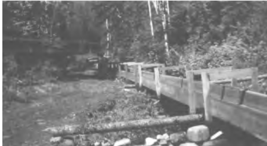
Ed Lundstrom flume's: water for gravel washing. PHOTO COURTESY OF BERNARINE STEDILE
