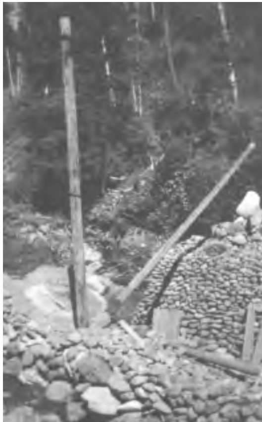
Gin pole: Ed Lundstrom placer claim at 15 mile on the Pend d'Oreille — circa 1920 to late 1940's.
