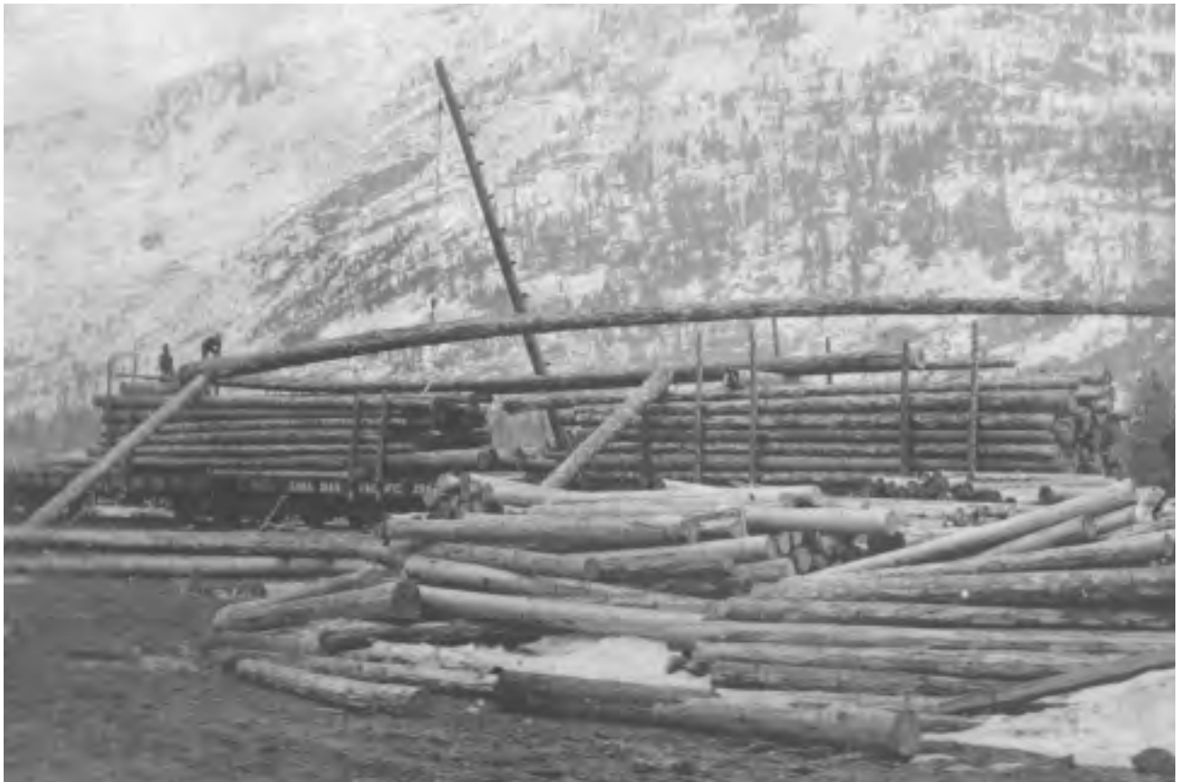
Cross loading long poles over 2 cars in Salmo — circa pre WWI. PHOTO COURTESY OF BERNARINE STEDILE
